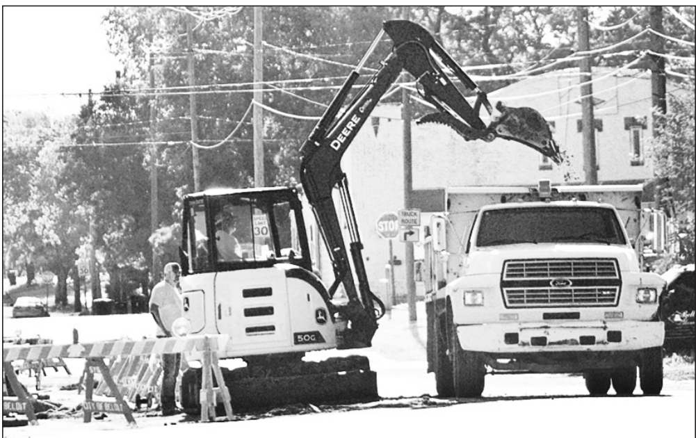
The Beloit City Crew is replacing a short stretch of water main on East South Street. They started on a Sunday to not disrupt business hours for others. There are a few more parts to go to hook into the hydrant, and then they will be finished.
