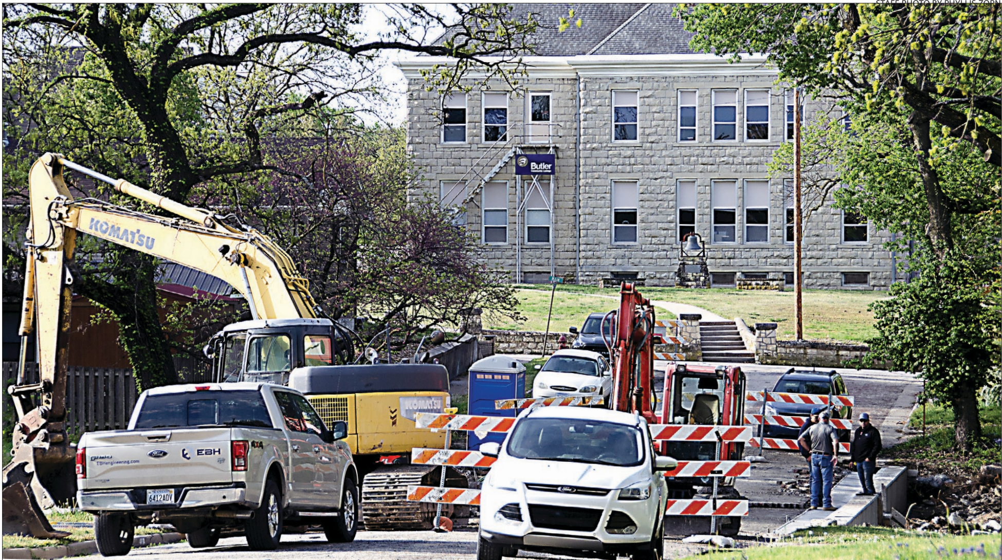
Workers are nearly finished with a long-delayed repair of Marion's Locust St. north of Main St. Erosion had left as much as eight feet of a box bridge under the street hanging in the air and endangered a retaining wall at the edge of the street. The state awarded a grant that would pay 70% of the $290,727 cost of repairs, plus new curbing from Lawrence to Main Sts. in October, 2022. Work began two weeks ago. Elm St. will be closed next week to excavate existing drainage pipes beneath the street and replace it with new pipes. Curbing also will be replaced. The same 70% grant for the Locust St. work includes the Elm St. work.
