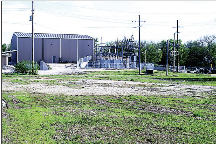
The Marion solar farm will be built north of the county transfer station and operational around June 2026.
