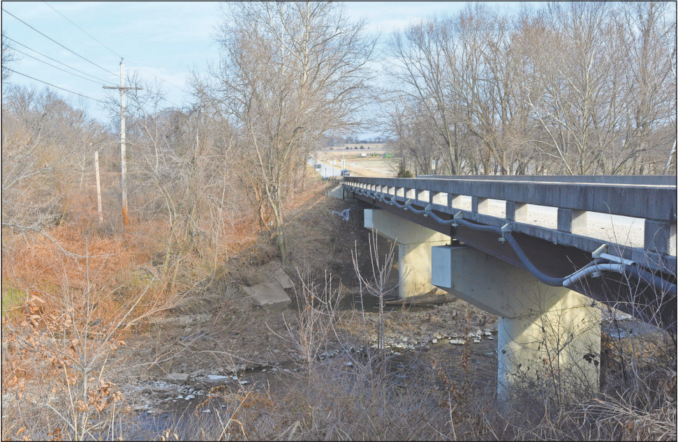
Streambank erosion along Wea Creek near 311th Street is threatening the stability of Paola’s primary waterline. The city plans to relocate the line to the south side of the road.
