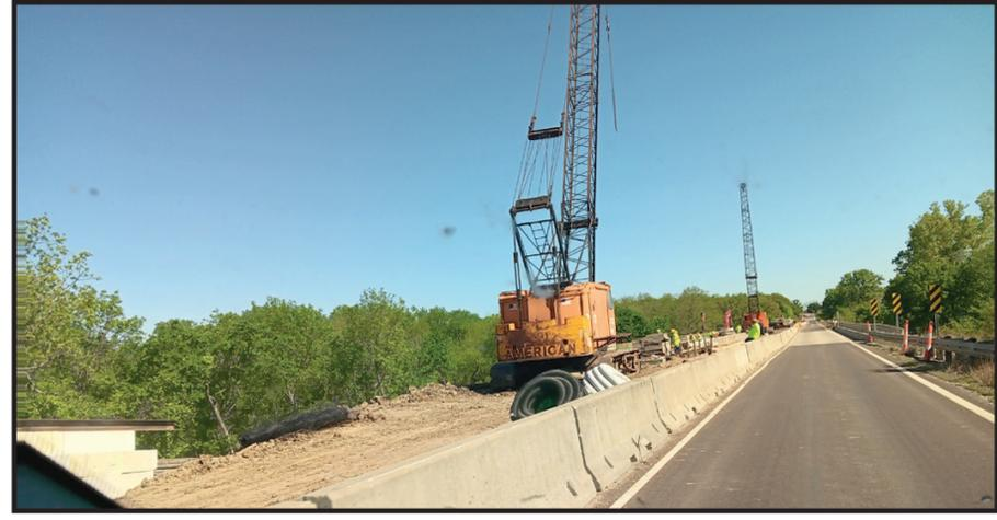
Work is ongoing on Cedar Creek bridge north of Toronto on Hwy 105. Forms have been set and are ready for concrete to be poured for the new side rail on Cedar Creek bridge north of Toronto on Hwy 105. Some concrete was poured last week on the columns underneath. Kathy Cummings/Citizen
