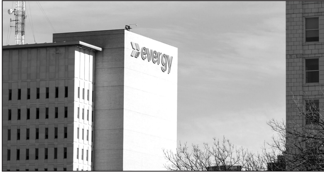
Evergy has approval from Kansas and Missouri regulators to build three natural gas plants and two solar fields. (Sherman Smith/Kansas Reflector)
