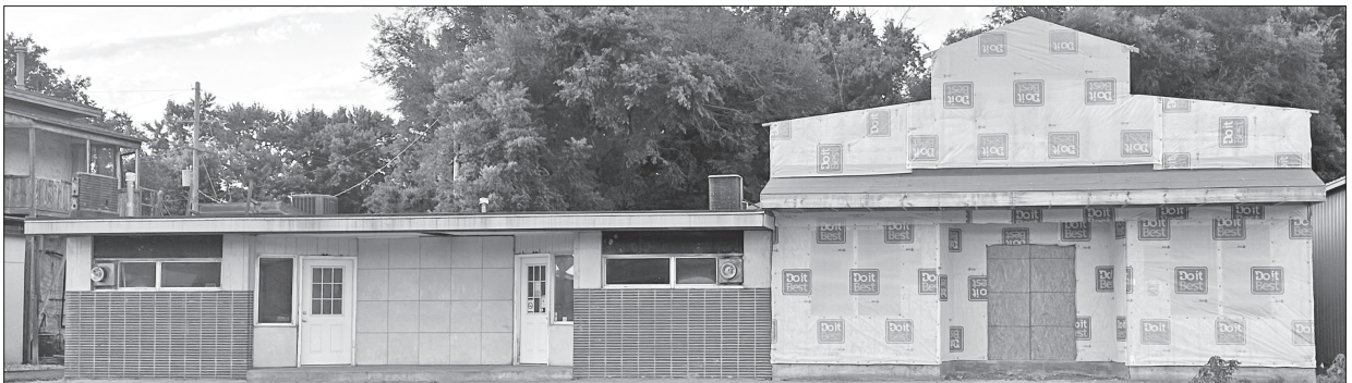
Passersby have been wondering what the status of 410 E. Main is since a stop work order was issued on March 13, 2026.
